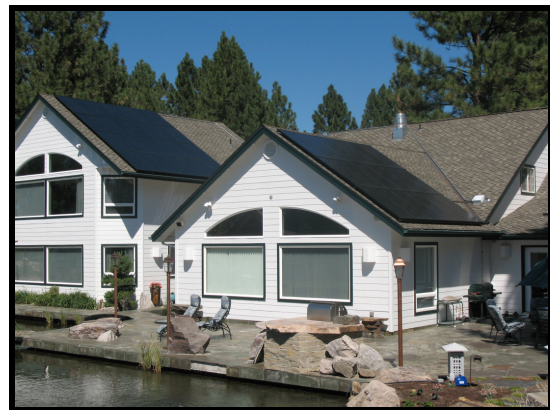
9.89 kW SunPower 205 Black Modules- Bend, Oregon
