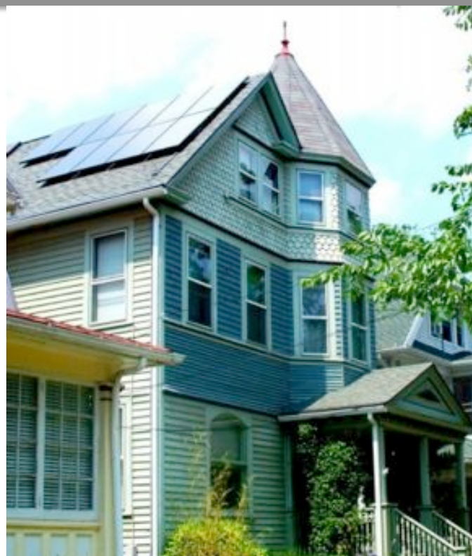
2.1kW Roof Mounted Solar Array
