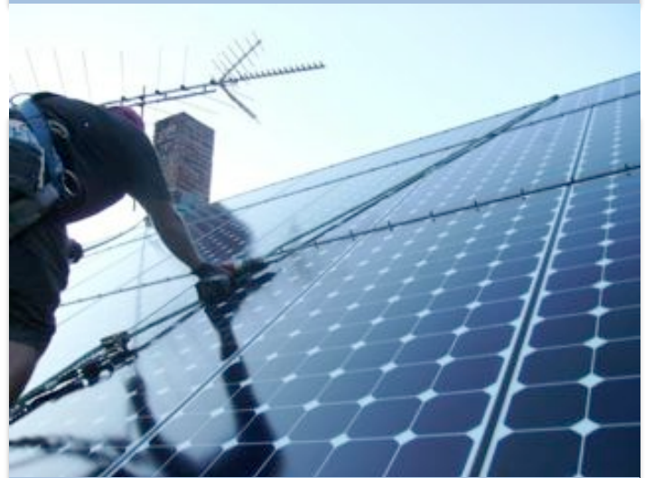
At Work On A 4.6kW Solar Array
