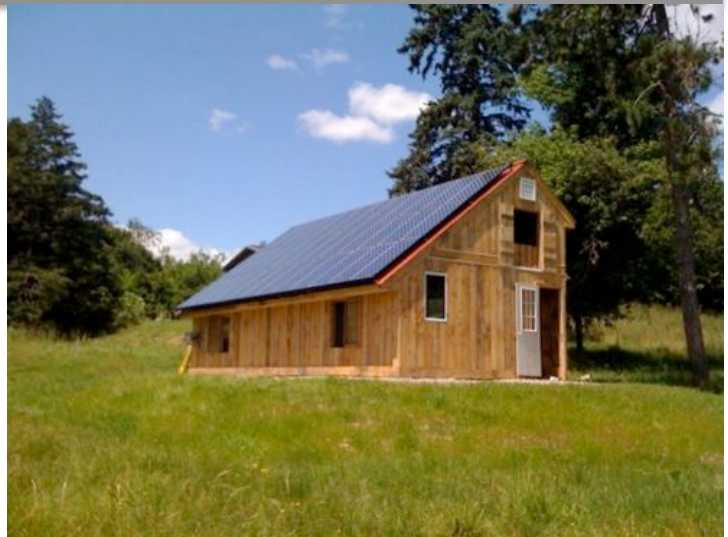
8.28kW Array Follows the Shading Rules of Thumb (see following page)
