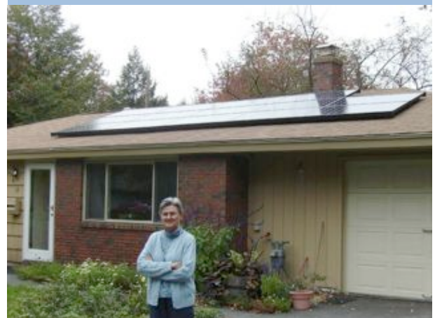
3.22kW Roof Mounted Solar Array
