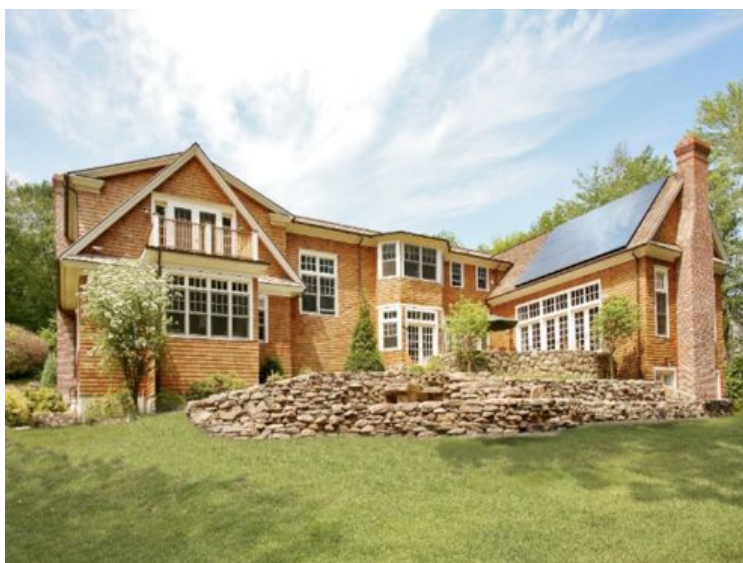
4.92kW SunPower Integant Award Winning Array
