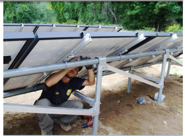
At Work on a 5.16kW Solar Array
