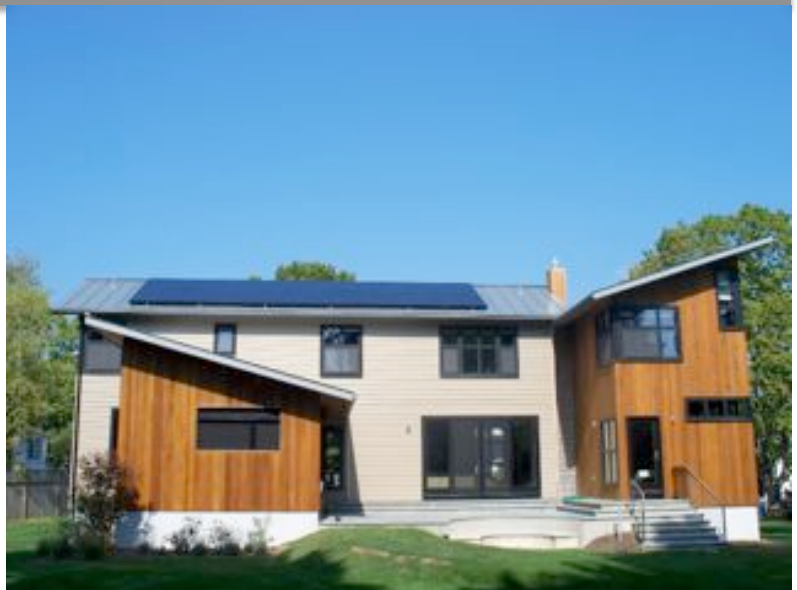
5.74 kW Roof Mounted Solar Array
