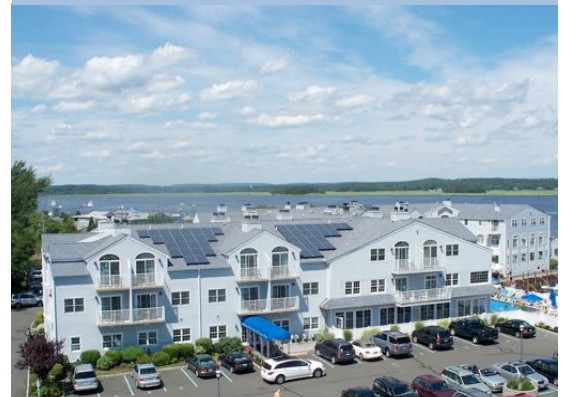
Saybrook Point Inn, 43.92kW Array
